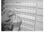
Record the splicing list on the card atta-ched on the front door. Check splicing, routing, storage and sys-tem status before starting the operation.
