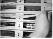
15. Completion of Work Pull out the patch cords toward the system through the reserved holes.
