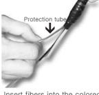
Leave 7cm from the Cable Sheath Insert fibers into the colored Prote- **4. OSP Cable Clamping** end and cut off the Tension Member ction tubes. Push the protection tubesecure the cable to the rear side of Leave 5cm from the Cable Sheath up to the locas tube and the sheat with a provided start band up to the loose tube end.
