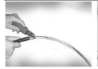
Remove plastic tape and dummy fillers. Clean the loose tube using jelly cleaner.
