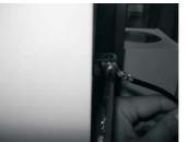
Connect Grounding wire to Ground Connect on the side of Grounding Terminal wire to Rack earth bar
