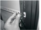
6. Fixing Splice Tray Fixed splice (STI 24-6) to the rear door with bolt (M3)
