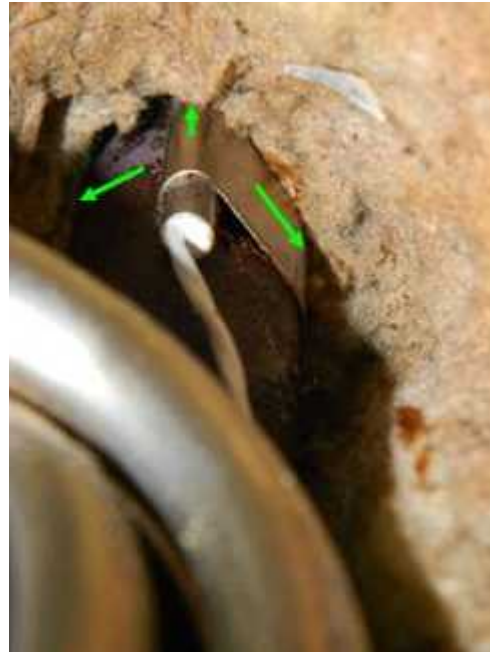
Fig. 6 Insulate RTD
