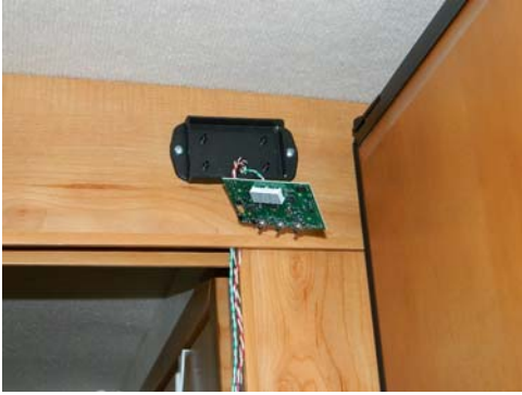
Fig. 7 Mount Housing & Route Wires
