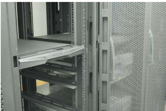
Figure 7. Push the LCD drawer until it is locked in the rack.
