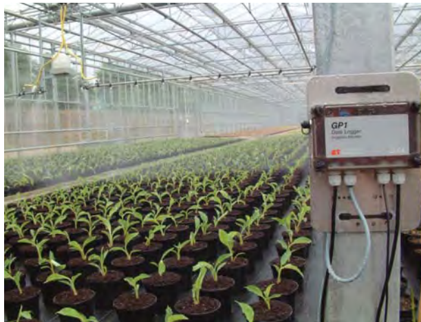
GP1 Data Logger controlling precision gantry irrigation within a glasshouse at Hillier Nurseries. The GP1 is connected to a single SM200 Soil Moisture Sensor installed in a representative pot.
