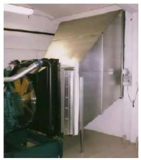
Under normal conditions, the air volume generated from the radiator's fan is enough to meet the requirement of the working room ventilation. The air inlet temperature of the engine shall be below 30 degree Celsius. If the air inlet temperature keep rising above 30 degree Celsius, the engine's output power will be reduced, and therefore fresh air from outside shall be introduced into the generator set's working room in a timely manner.
