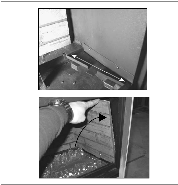
Figure 8.16 Install left or right side panel. Place in lower channel and rotate into place.
