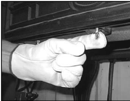
Figure 8.12 To remove the face, loosen the thumb bolt beneath the ashlip.
