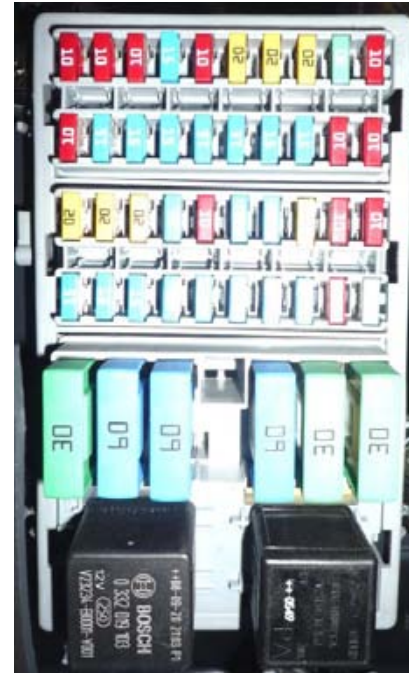
Fuses types and fuses control unit
