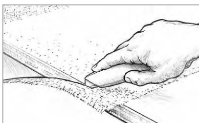
Figure 26 Trim excess cloth after the epoxy gels.
