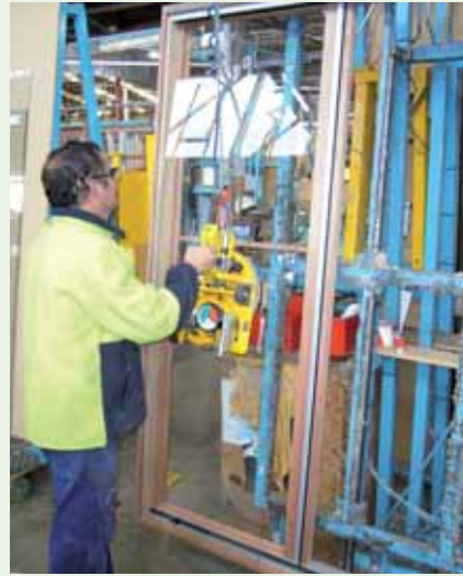
Vacuum lift for glazing windows
