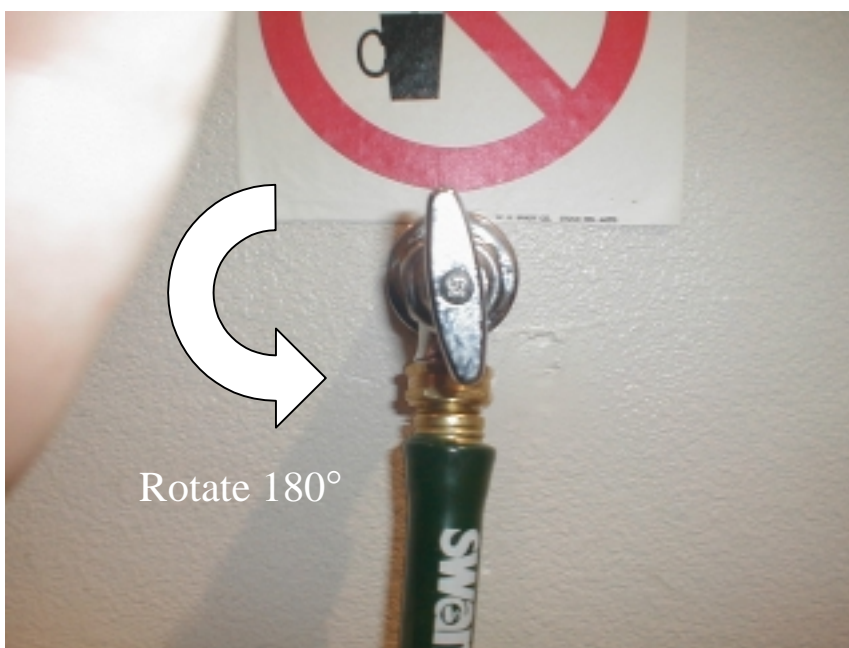
Figure 26. Water Coolant Valve Turning 180°
