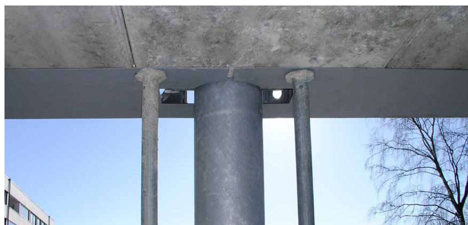
Figure 6. Propping DELTABEAM.
