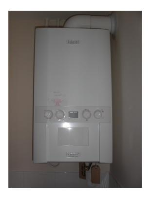
From this, hot water is circulated to the radiators in each habitable room via distribution pipework located under the floors. A programmeris situated in the hallway which allows you to control your hot water and central heating.
