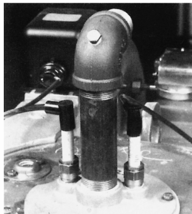
Flame rod fit with 4-30HP Boiler
