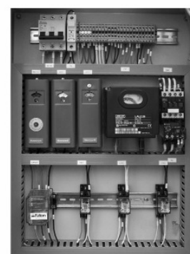
80-150HP Fuel Oil(Left) Gas(Right) Siemens series Control panel
