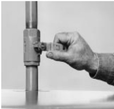
1) Shutting off the water outlet valve
