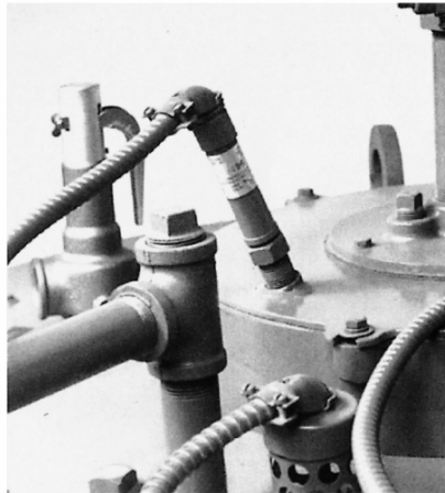
UV Scanner fit with 20-150HP Boilers
