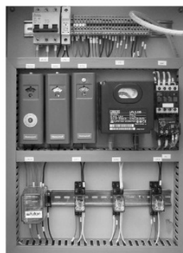
80-150HP Fuel Oil(Left) Gas(Right) Siemens series Control panel
