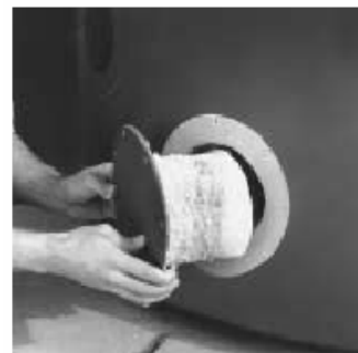
4) Remove all soot from the top, and from the clean out plugs at the bottom with a vacuum cleaner.
