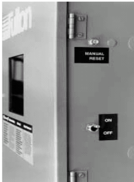
Place feedwater pump fused switch in the “on” position.
