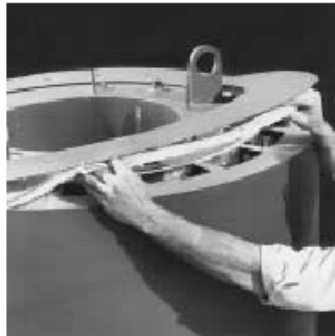
2) Wire brush flue passage
