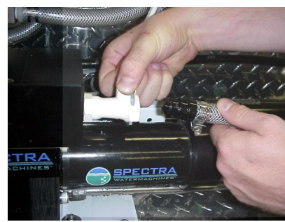
Connecting brine discharge service hose
