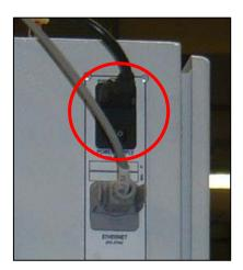
The industrial Ethernet socket is of type VARIOSUB-RJ45. The recommended Ethernet cable is of type KVL-ETN.
