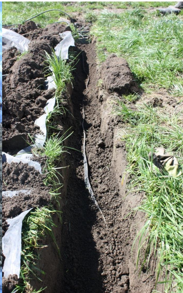
Top sensor being installed to 25mm at the deep end.
