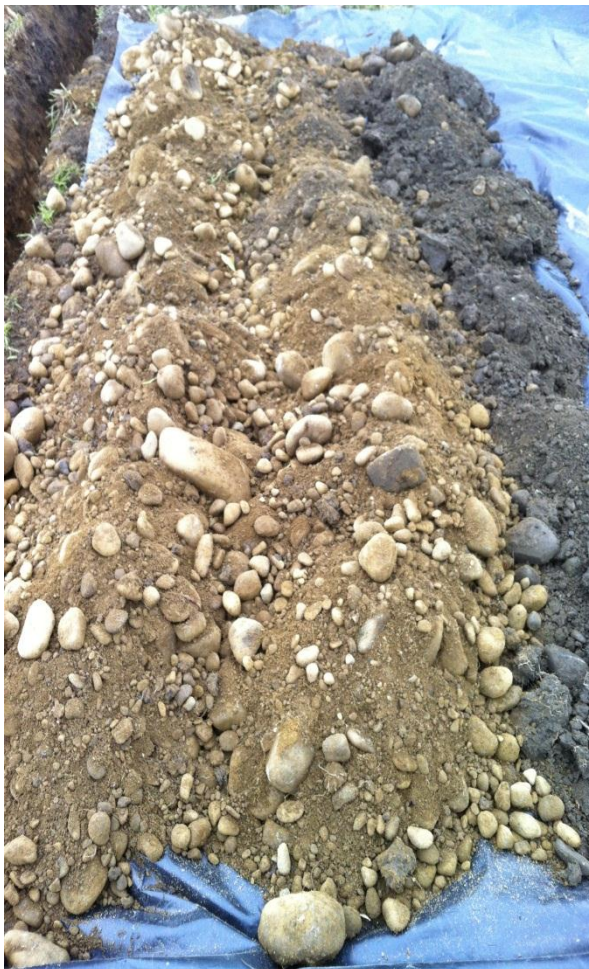
Soil removed and placed in three layers.
