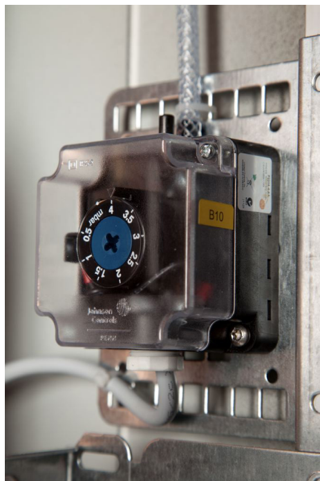
Air filter clog switch
