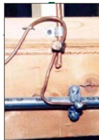
Install bonding jumpers around conductive material.
