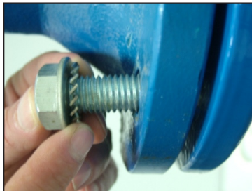
STEP 5 Insert flat washer and serrated washer on bolt - use the correct washers per bolt size (M16 or M20 respectively). Insert the bolt in the hole of the pipe's flange - do not insert on meter's flange.
