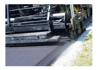
Each paving machine manufacturer has their own unique screed and screed extension design. Our road safety edge products and center lane jointing products are designed to attach to most standard paving machines by simply drilling two holes in the screed (or screed extension).
