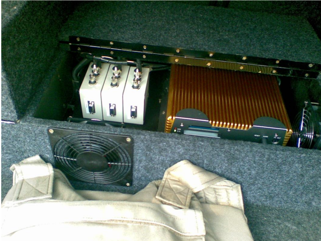
Figure 3.2: a typical installation
