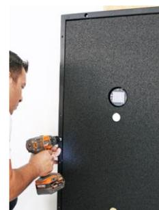
1. Place panel #P1A on the lower left corner of the plywood wall.
