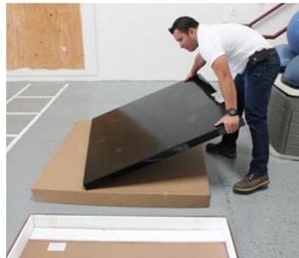
13. Open and remove the lids of the boxes of the station panels and lay them in front of wall lying face up in their boxes.
