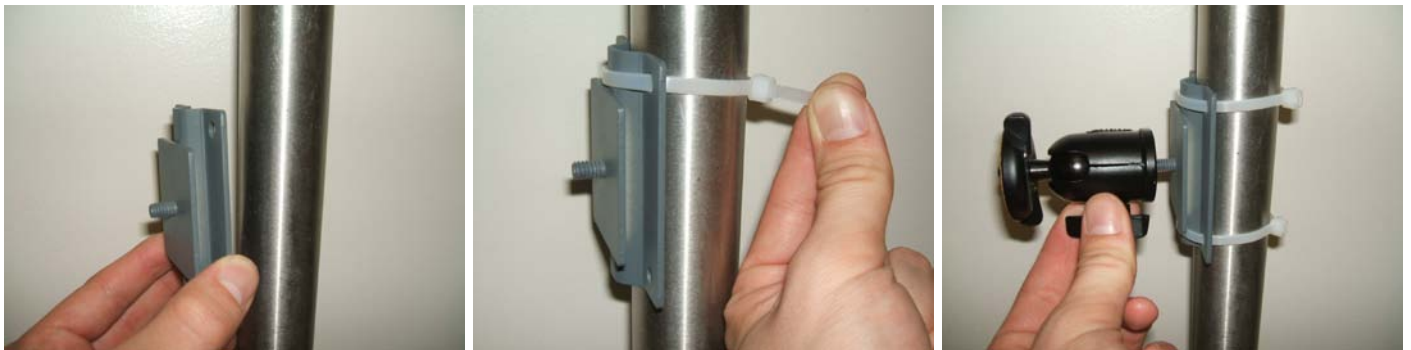
Figure 15: Installing Mini-Thermal Camera Bracket to Pole
