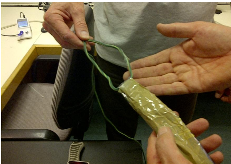
Figure 4: Draw-string through the loop at the end of the fiber-optic cable
