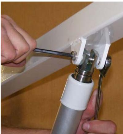
Remove the shipping strap and all packing from the LINEAR ACTUATOR. Connect the LIFTING ARM between the MAST and the ELECTRIC LIFTING RAM as shown in the figure above. Tighten NYLOCK NUTS (2) until snug as shown in PHOTO 2. **DO NOT OVER TIGHTEN!**
