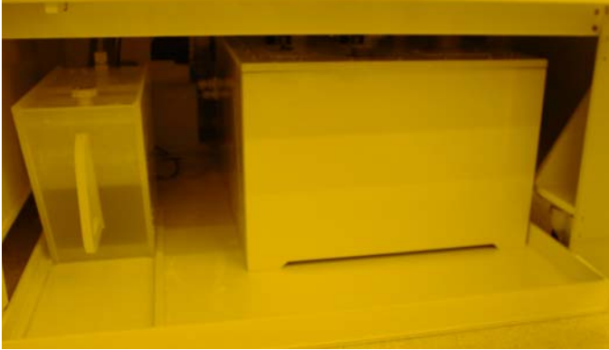
Figure B4. Under Deck caustic tank (left) and neutralization tank (Right). The caustic tank will slide out enough to fill through the lift-off lid at the front top.
