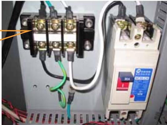
Fig. 4-7 Install the O shaped Cord to Terminal Connector
