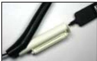
Threading the armor with cable.
