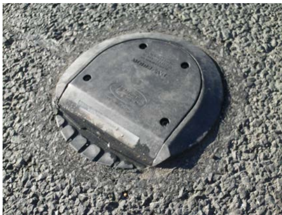
Figure 1: Example of properly installed 10" composite baseplate
