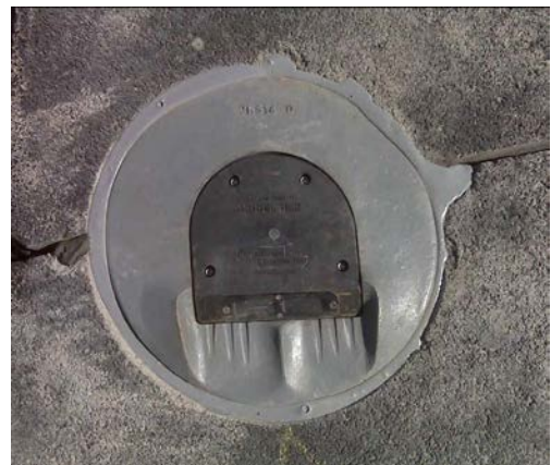
Figure 1: Example of properly installed 14" baseplate in a snowplow region
