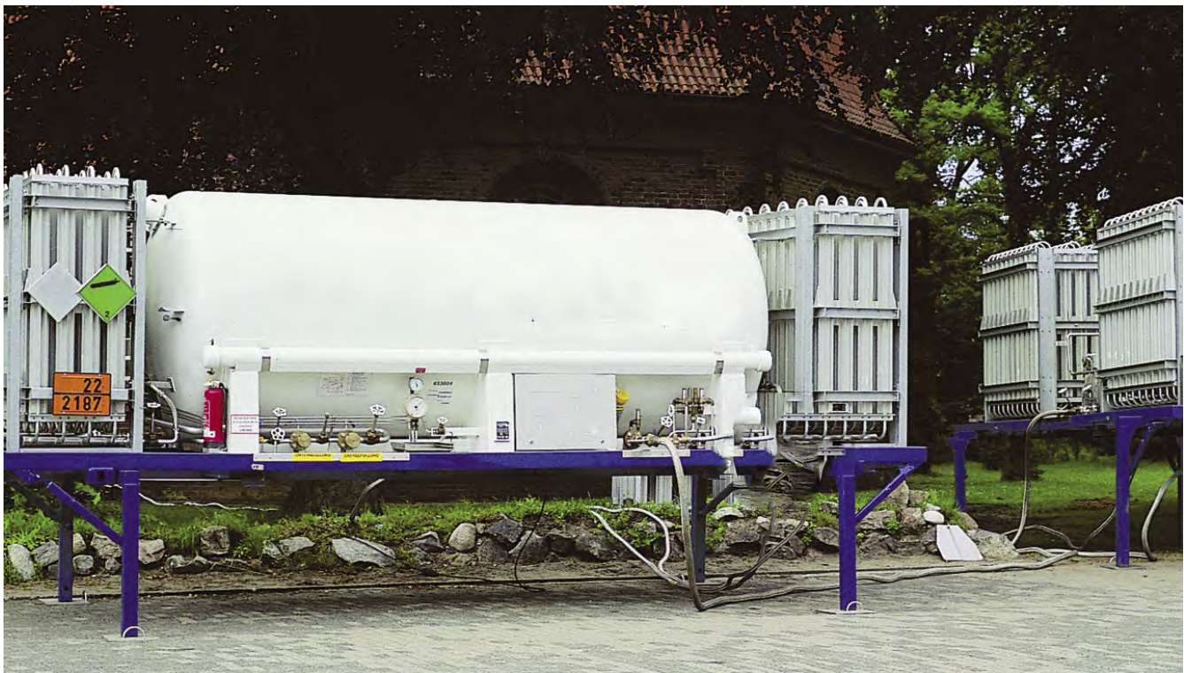
Picture 6: Tank trailer and mobile evaporator
