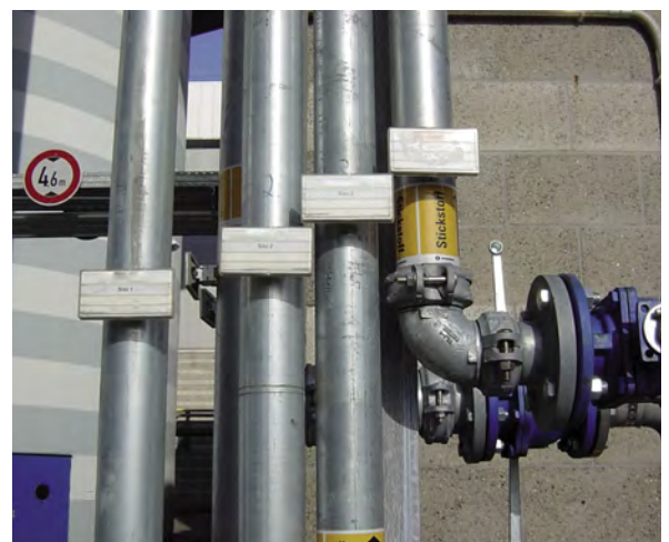
Picture 10: Inert gas feeding through pre-installed pipes
