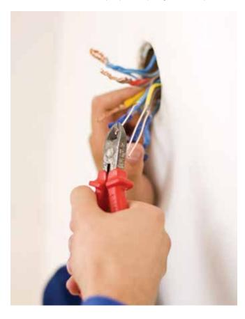
a copper joint. Corrosion is another major risk of using other metals and alloys in wiring. Commonly called a 'noble metal', copper is not susceptible to galvanic corrosion when connected to non-copper metals. It effectively resists moisture and humidity driven corrosion that can destroy other wiring systems, reducing the risk of power outages, system failures and fires. Copper wiring typically does not require the use of conductive greases at its connections, and torque is not critical.
