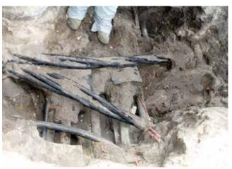
Figure 1: Local heating caused by cable installation configuration. (Substation exit cable photo courtesy AECOM).
