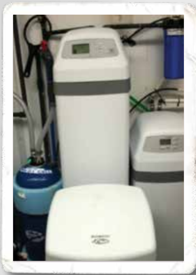
PICTURE 7. REVERSE OSMOSIS WATER METER
