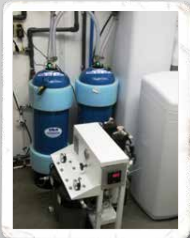
PICTURE 8. DEIONIZING TANKS FOR WATER SYSTEM
