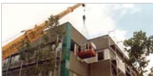
crane delivery of h/p/cosmos saturn®
