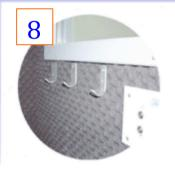
Place the hold-ups for the accessories that the patients are going to use where desired (always inside the booth), having in mind this position must not bother the patient and must allow to perform the audiometry. They should be lined up and
