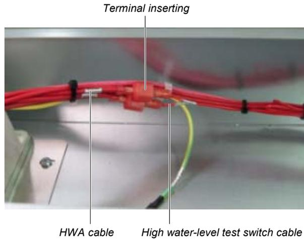
**Figure 2-33** Connecting the corresponding cable terminals of the high water-level detection switch and the HWA cable terminal
