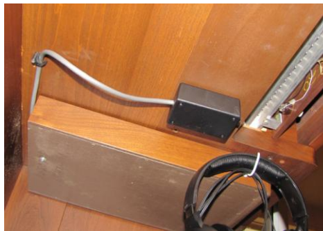
Photo # 3b: Jack Box mounted and covered.
