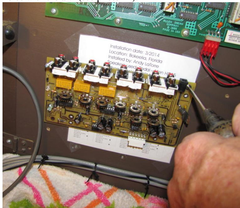
Photo #4: Mounting the HMA circuit board. Using awl to mark location of right side mounting hole. The left side screw is temporarily used to hold board up. Note the towel below to prevent dropped screws from doing any damage.
