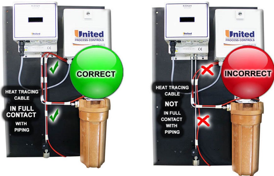
Figure 8 Heat trace cable installation
