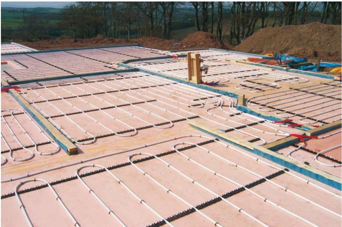
Floor heating needs to be designed into the building structure and can be fitted early on in the building schedule.
