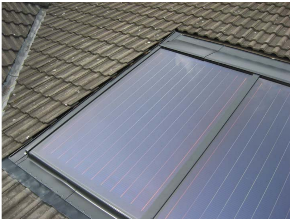
Figure 13: Panels being retrofitted to tiled roof
