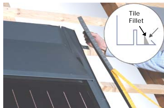
Figure 5: Side flashing for tiled roof
