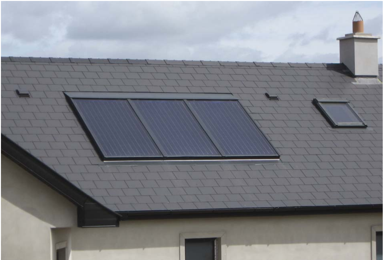
Figure 8: Completed installation on slate roof
