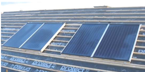
Figure 3: Collectors fixed on roof before installation of flashings
