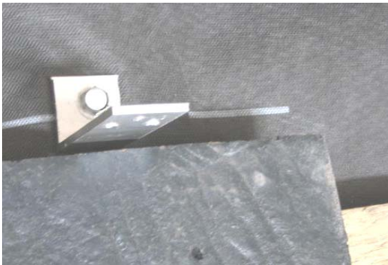
Figure 2: Fixing bracket on lower side ready to take collector
