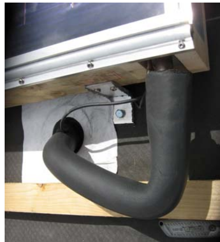
Figure 4: Felt grommet where pipework penetrates felt
