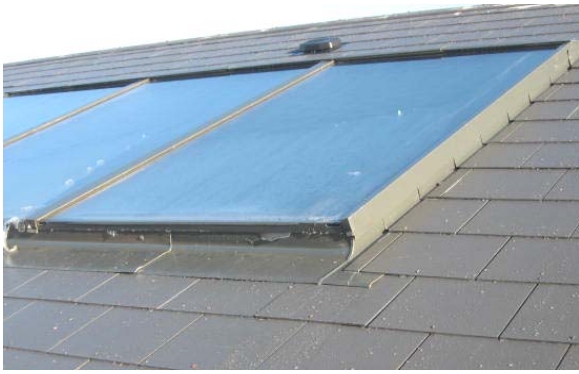
Figure 6: Finished flashing kit on slate roof
