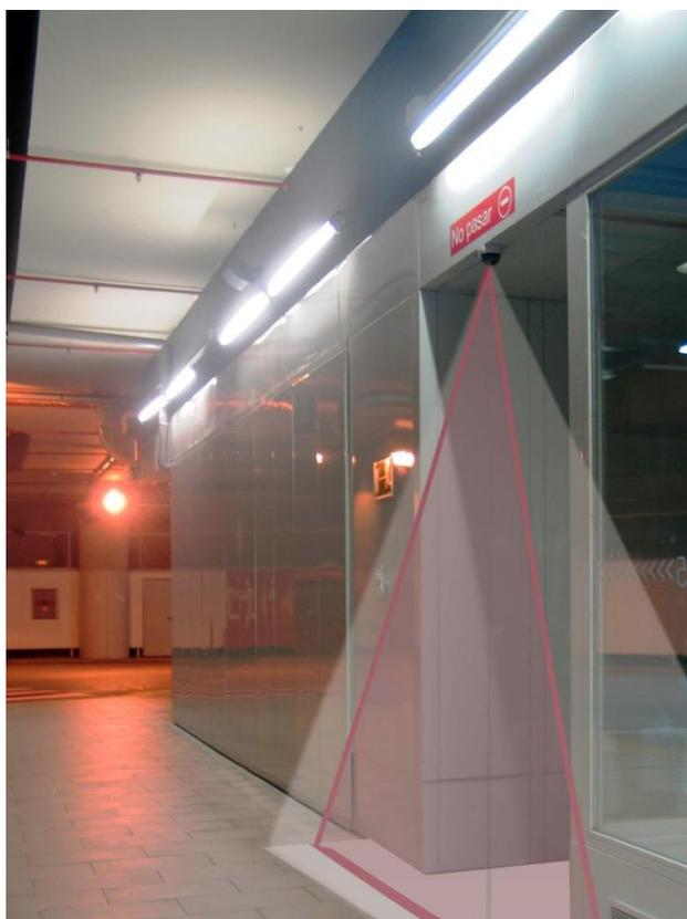
Fig. 1 – Peco camera installation
