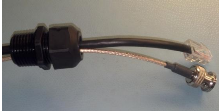
Figure 11: Tighten Gland Nut & Terminate Cables
