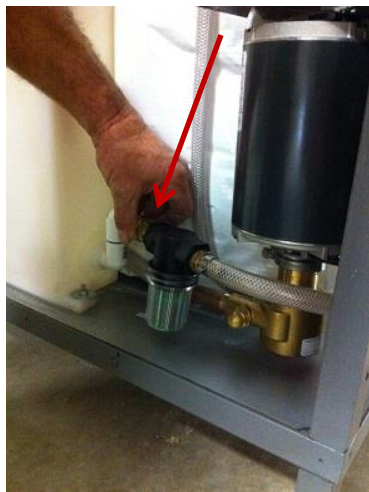
Unscrew Brass Disconnect
