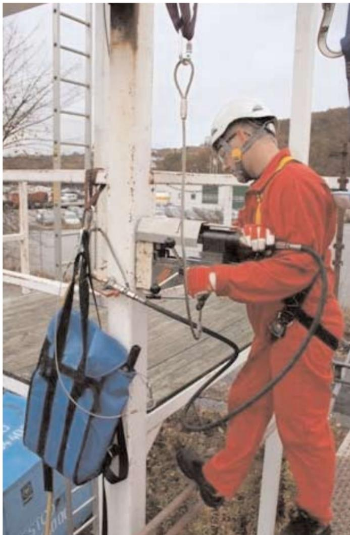
Methods for securing heavy tools and hand-held machines for use at height have not been adequately defined. In view of the major potential for serious damage if such tools or machines fall, it is important to have clear guidelines.
