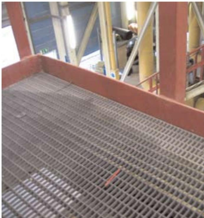
In many cases toe boards have either been lacking completely or the gap between the toe board and the deck has been big enough to allow objects to pass.
