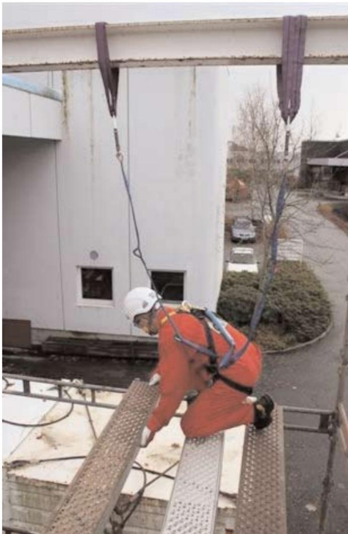
In work at height for which anti-fall equipment is mandatory, the necessary expertise is required to ensure safe working conditions.
