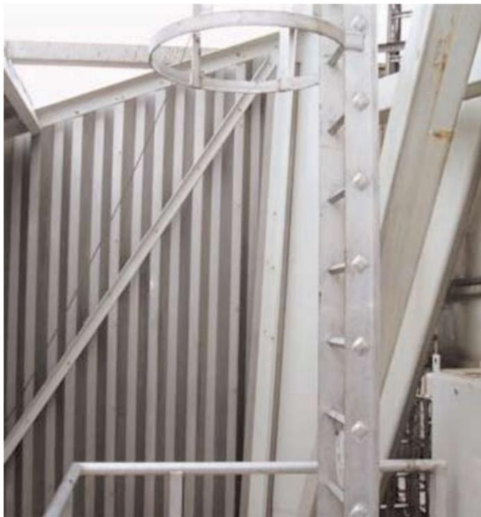
Many cases have been found of damage to ladders and safety cages as a result of collisions with mobile equipment. In addition, cracks have been found in safety cages, especially in derricks.
