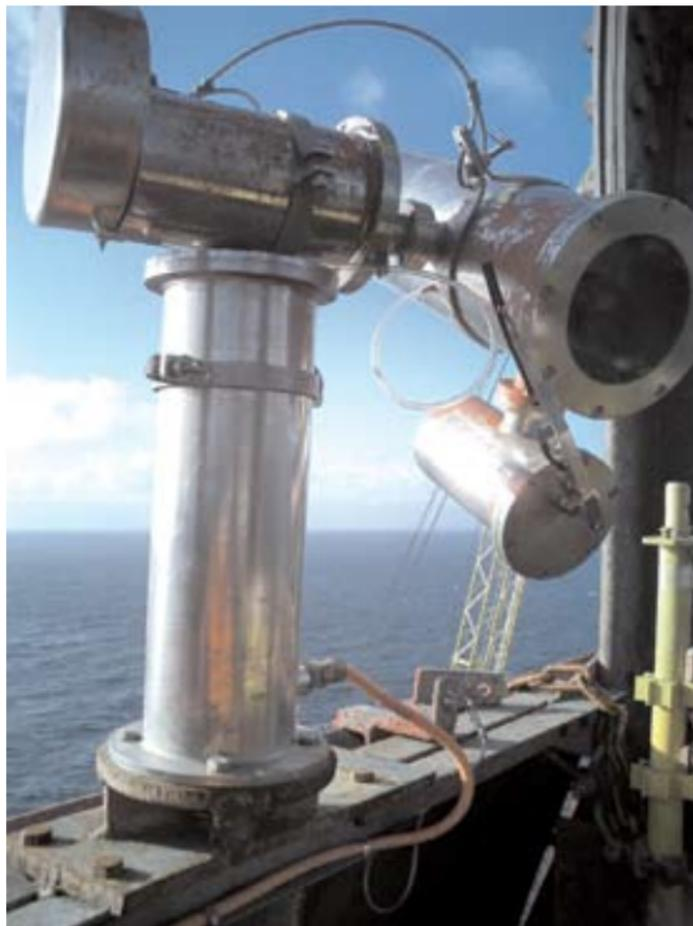
Many CCTV cameras are inadequately secured. There have been several cases in which both the camera and the control unit have come loose from the brackets and fallen on to the deck. The total weight may be as much as 50-60 kg and there is a significant risk of serious injury/damage.
