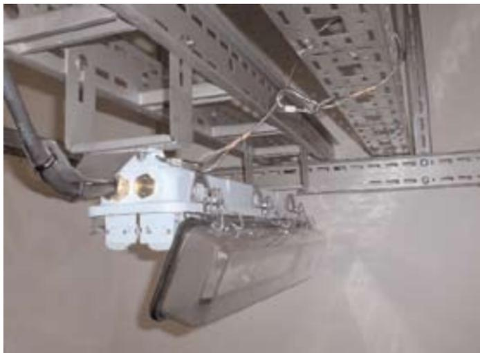
Several types of light fittings found on our facilities are inadequately secured against falling. There have been several serious incidents in which both the cover and the casing of the fixture have worked loose and fallen down.
