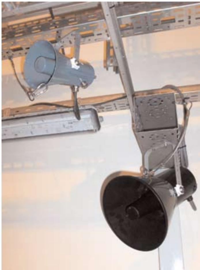
There have been several cases where we have discovered loose screw connections between loudspeakers and attachment braces/brackets.
