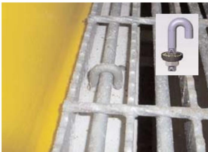
At present there are a number of different ways of fastening grating to underlying structures or frames. As a result of vibration and defective locking of fastenings, there is too much loose grating and too many fastening clips of various kinds are loose or missing.
