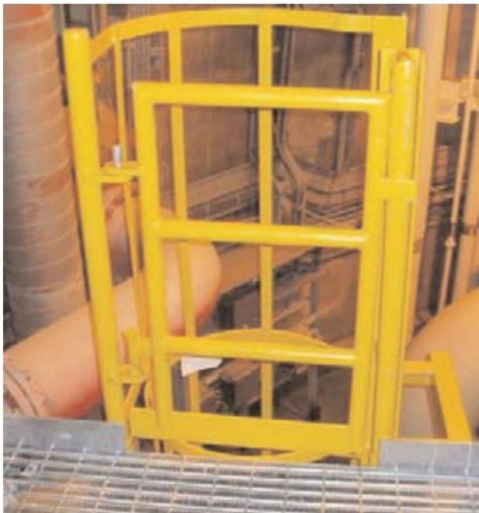
Many swing gates have been found to have hinges with neither the necessary quality of material nor the design strength to serve their intended function over time.
