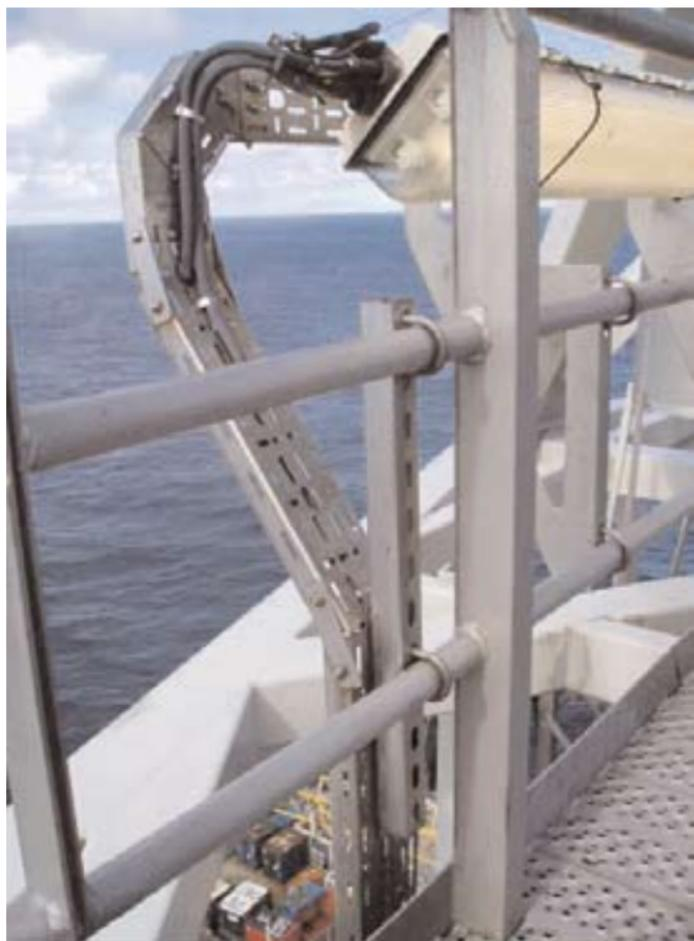
Many instances have been discovered of loose nuts and bolts in the joints and fastenings of cable ducts (electro-steel), probably as a result of vibration and/or faulty installation.
