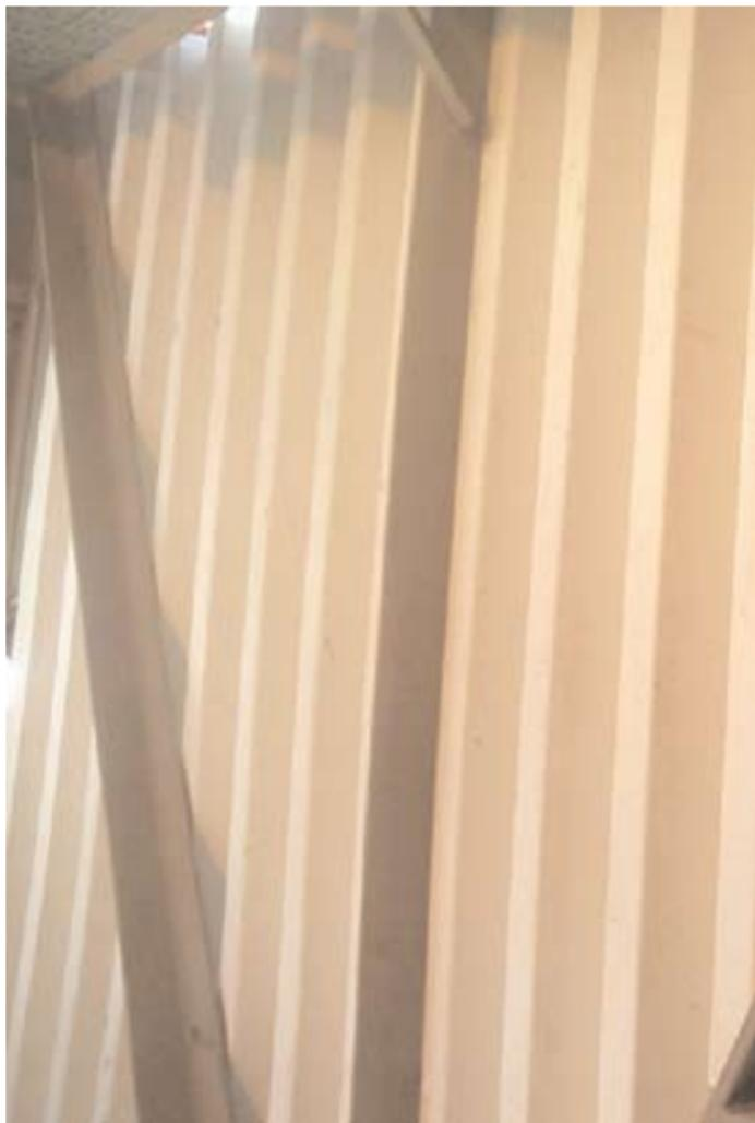
Many cases of damage and loose panels have been found in wind walls. This is presumably due both to faulty installation and to external factors (collisions with mobile equipment and exposure to wind and weather).
