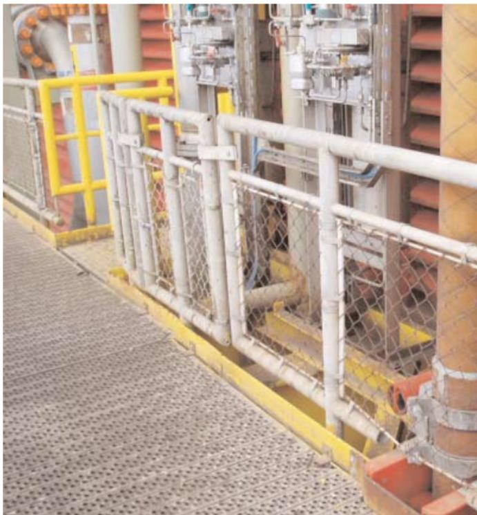
Major defects have been discovered on railings, in particular collapsible and movable railings. We have found recurring instances of railings that are inadequately inserted into the fastenings as a result of external impacts, causing disparity in the size of the holes for inserting the securing pins.
