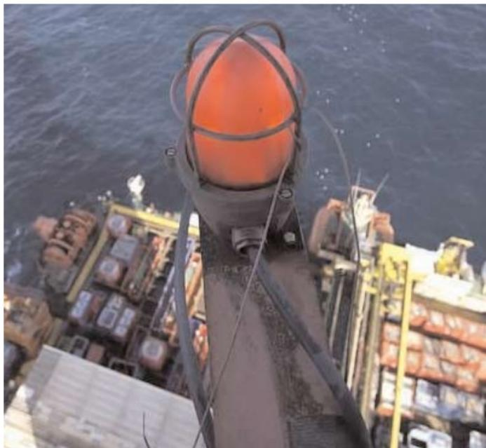
Several types of navigation light used on our facilities are inadequately secured against falling.
