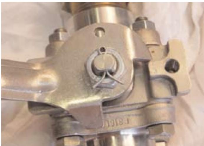
Many cases have been discovered where valve wheels and valve handles for manual stop valves are not adequately secured.
