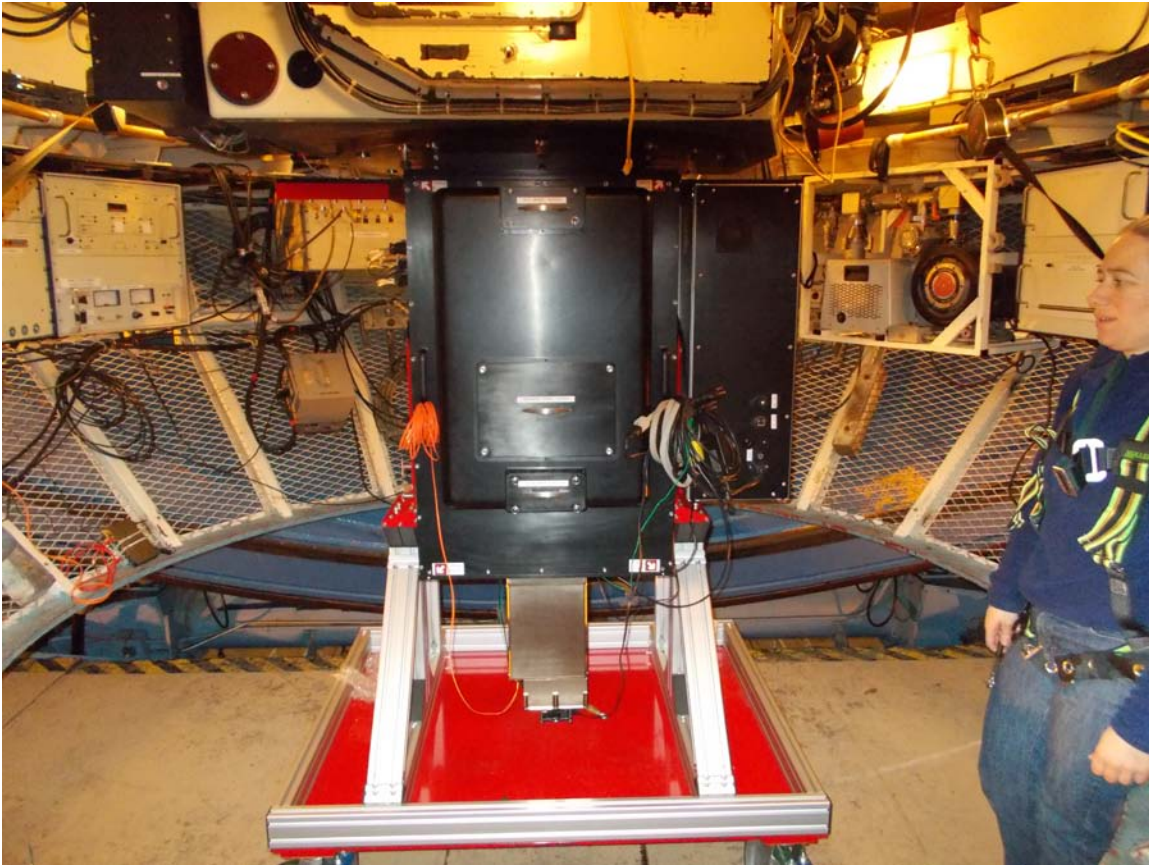
Figure 4: KOSMOS on handling cart, on mirror lift while being installed on the rotator. The view is from the direction of the cage door; note the access hatches visible from this position.
