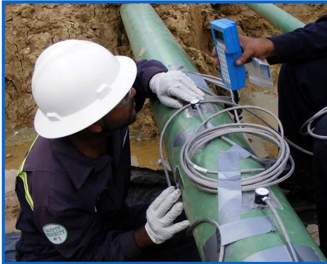
Figure 4.8 – Located the best spot for mounting with the epoxy.
