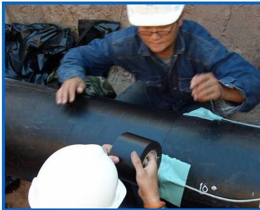
Figure 4.7 – Different transducers affixed to pipelines and pipe repair being applied.
