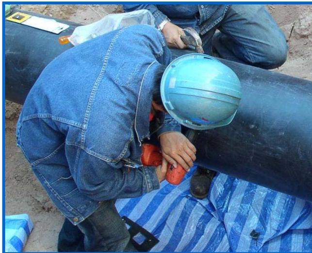
Figure 4.3 – Sanding the Pipe Surface.
