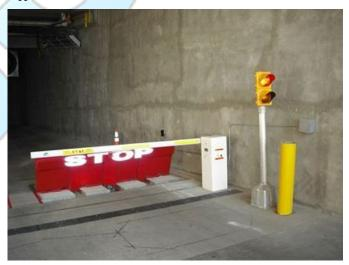
After Sensors send a call to IOBridge.Net, system will proceed on Indicating by Traffic lights or barriers to prepare the vehicle driver enter or leave the weighbridge.
