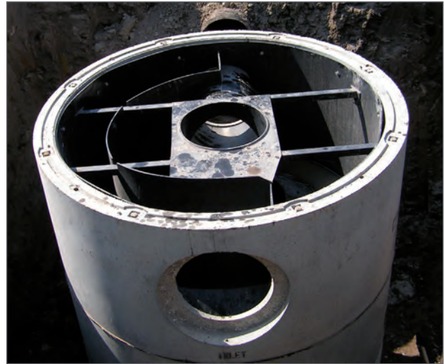
High Density Polyethylene (HDPE) internal components fully fitted into a reinforced precast concrete chamber.
