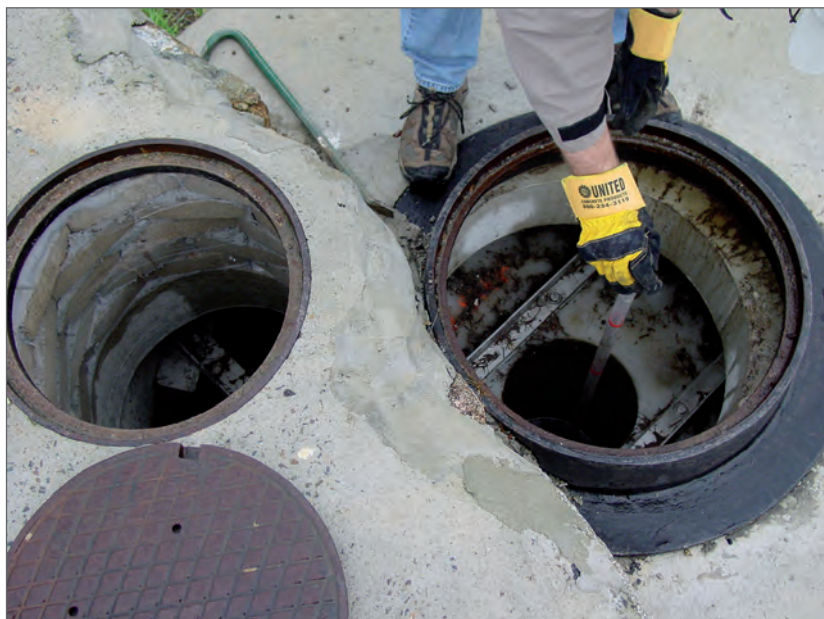
Depth Gauge Measurement of Captured Sediment
