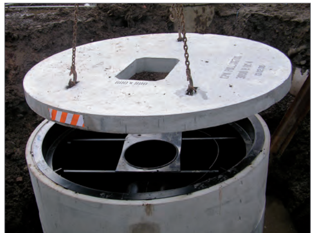
Cover slab being craned into position.
