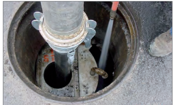
Cleaning of Internal Components and Pollutant Removal via Vacuum Tanker Hose.
