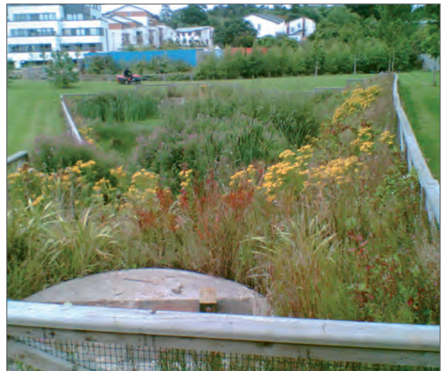
The completed, attenuation pond. The Downstream Defender® manhole can be seen in the foreground.
