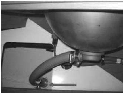
Washbasin draining Head version - aft
