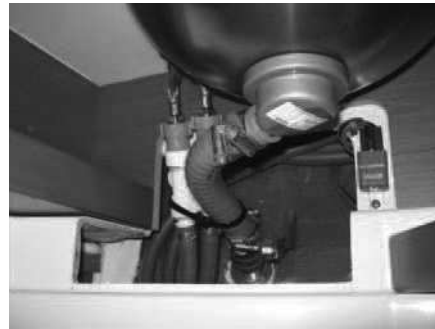
Washbasin draining Head version - forward
