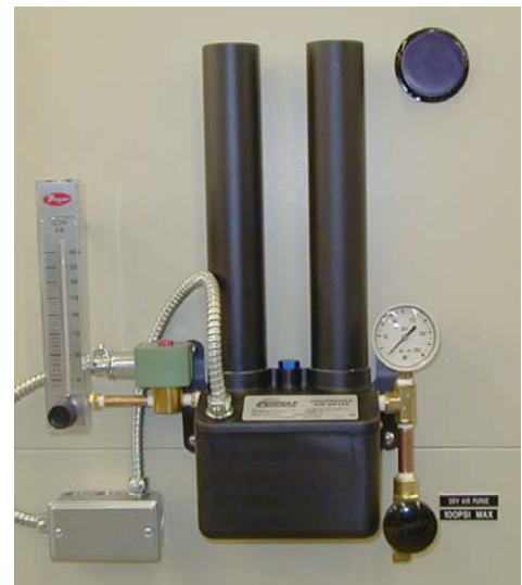
Heatless Desiccant Dryer
