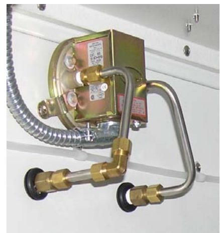
AIRFLOW SWITCH
