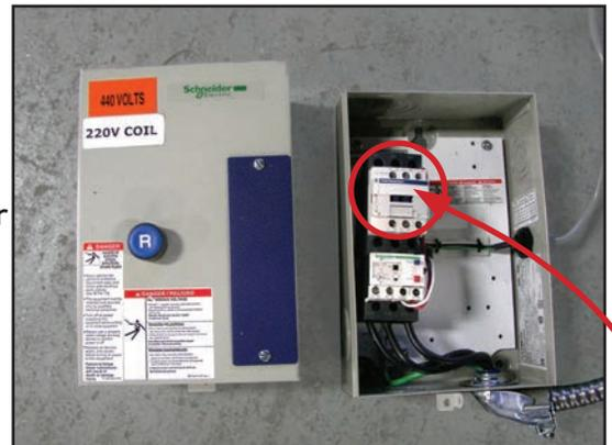
You will need to have the electrician connect AC power (**220 or 440VAC**) as specified on the unit **here** to the Motor Starter.
